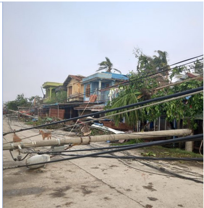
Electricity infrastructure damaged in Sittwe. Photo: IOM Myanmar
