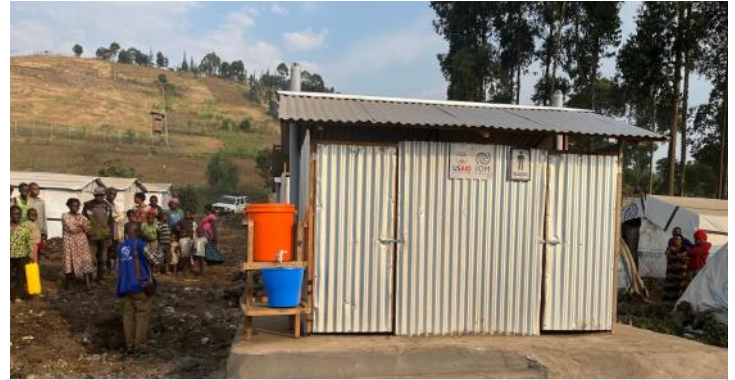
Newly constructed latrines in Lac Vert/Bulengo site, July 2024 @IOM 2024
