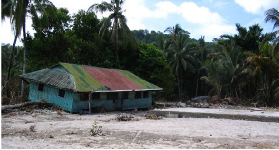
A house washed right off its foundation by the 2 April 2007 tsunami in the Solomon Islands. © Scientology VM Disaster Response Team, 2007
