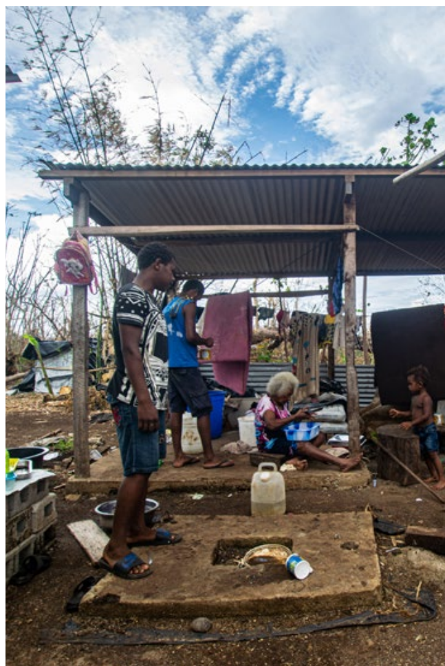
Families who moved to Santo during the evacuation of their home island, Ambae due to the Manaro eruptions, waiting for their roofs being repaired after TC Harold. April 2020, © UNICEF/UNI324730/Shing
