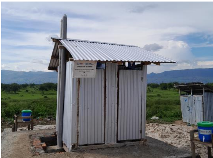
Latrines constructed in Tchomia, Ituri © IOM DRC 2023
