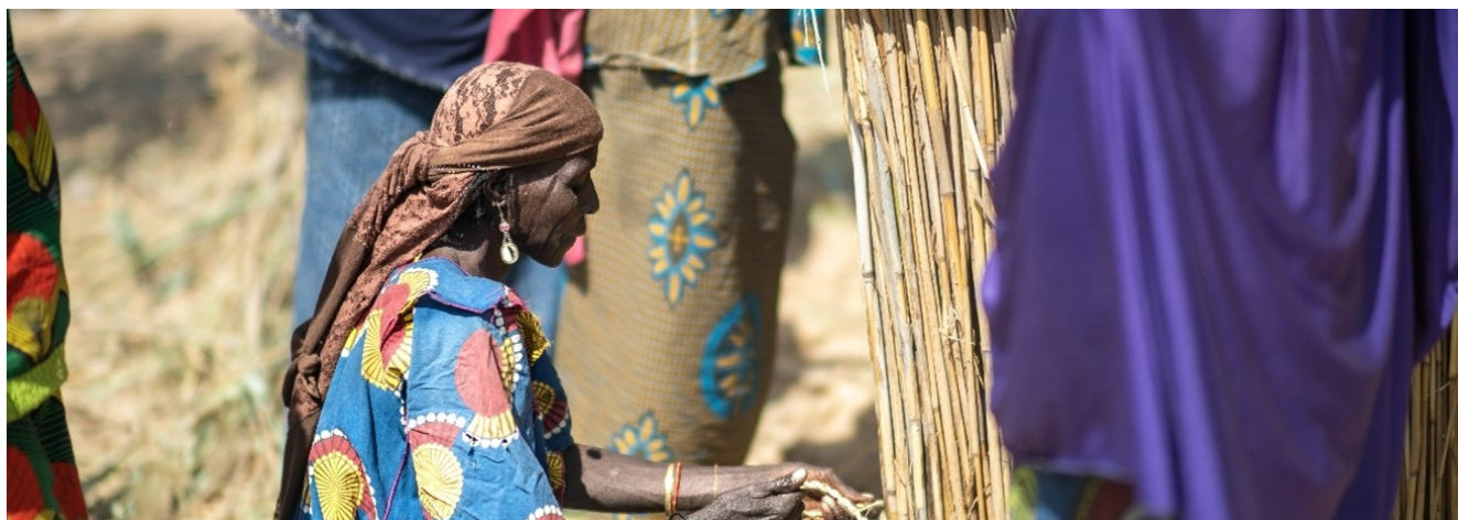
Lake Chad province, Women working on the construction of straw shelters. © IOM Chad /Andrea Ruffini, 2020
