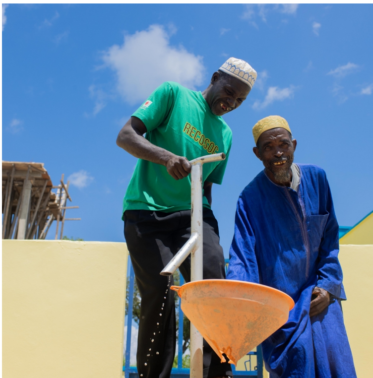
The installation of the human-powered water pump in the village of Massala Barala supports border populations in addressing the challenge of limited access to clean water ©IOM/Mohamed Aly Diabaté 2022
