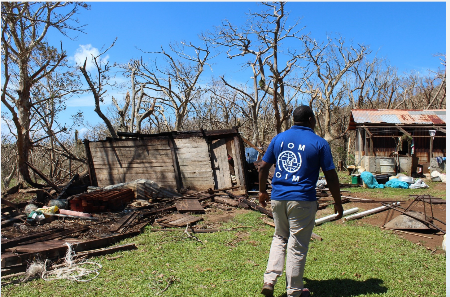
Wrecked cooking area in the village of Emae after Cyclone Pam. © IOM 2015/ Joe Lowry
