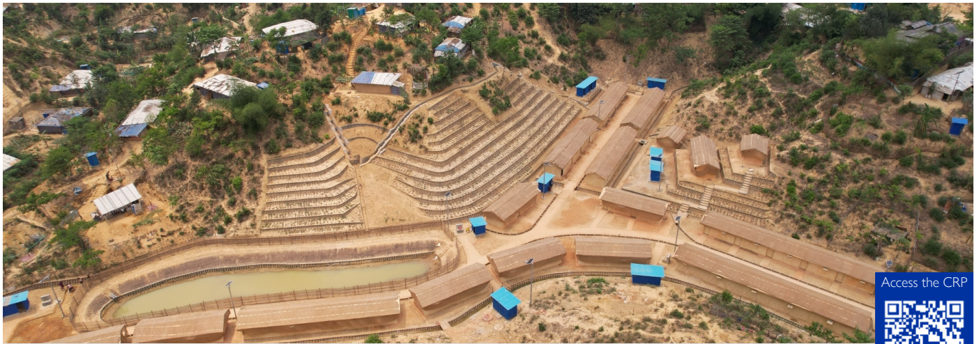
IOM's Innovation Valley in Camp 20 piloted 51 shelters and site development constructions using Lime Stabilized Soil (LSS) © IOM Bangladesh 2024 / Hossain Ahammod
